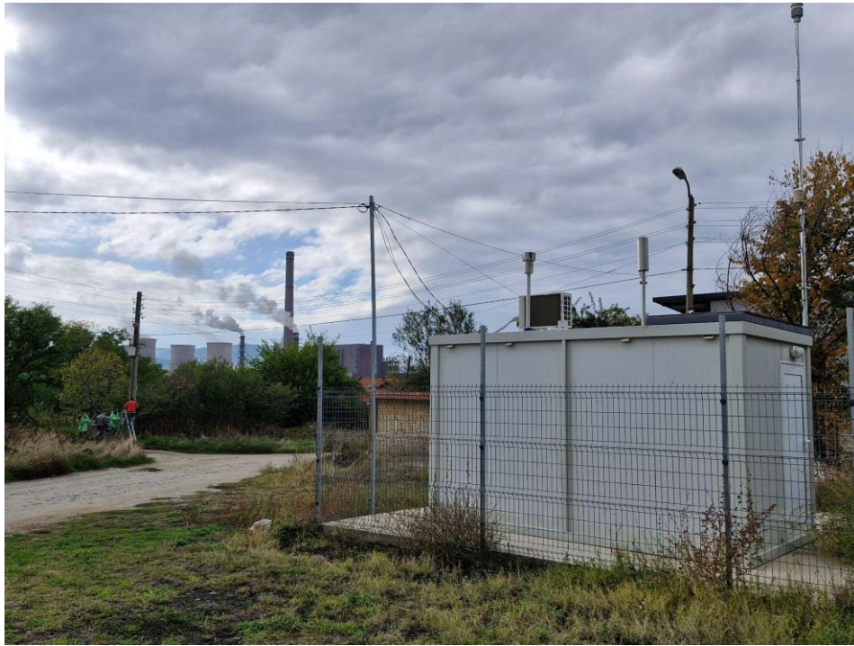
Figure 5. “AMS Golemo selo” (front right), Greenpeace team installing the DTs at location near the AMS (bottom left) and CFPP “Bobov dol” (at the back)
