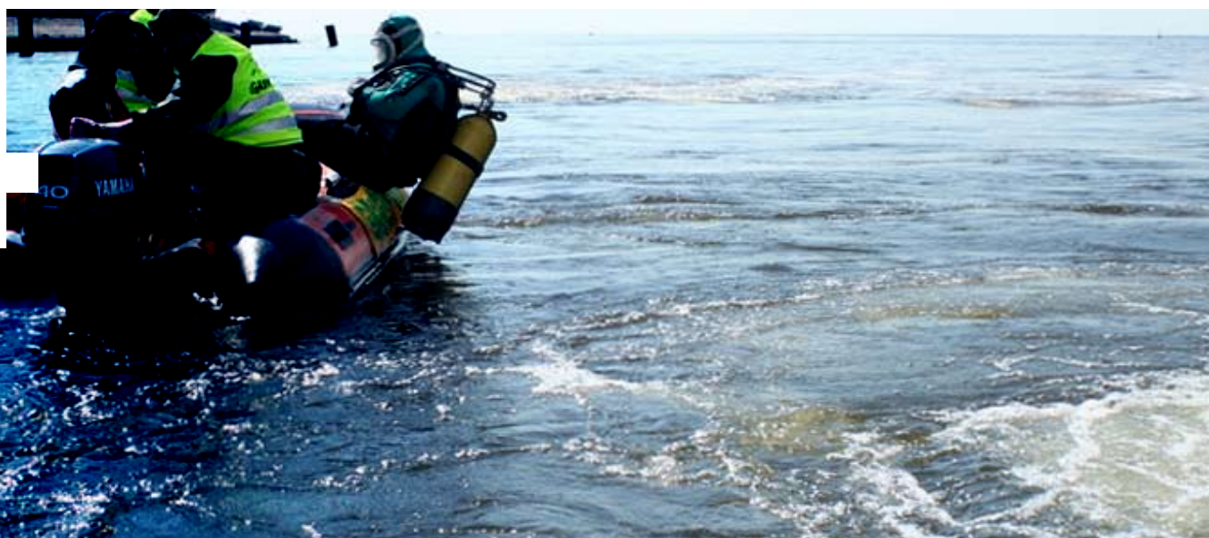
Underwater effluent dispersing pipe of Central WWTP, located at Nevskaya Guba, Gulf of Finland, St-Petersburg, Russia, 2007. © Greenpeace
